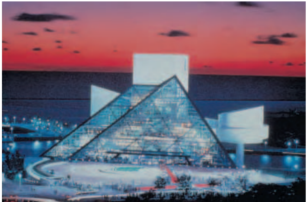
▲ FIGURE 14.16 This building must hold an extensive collection of artifacts while expressing the spirit of rock-and-roll. Do you think it serves its purpose?
